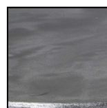
Concrete Steel Base
